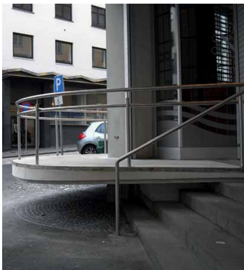
The ramp is finished. Note the tactile surface under the ramp (idea provided by the NABP). Photo: Bergen municipality
