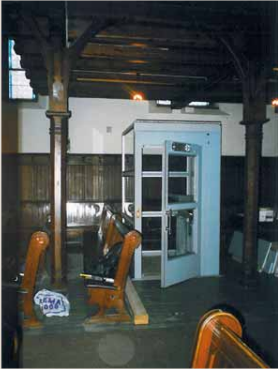
The lift being built before being covered by wooden panelling (incorrect representation of the colour)
