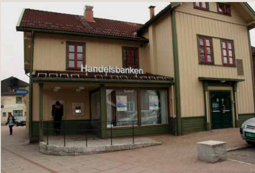
The Veiberggården building in Jessheim. Access to the ATM is ensured via a low ramp that makes use of the difference in height in the ground around the building. Photo: Ullensaker municipality
