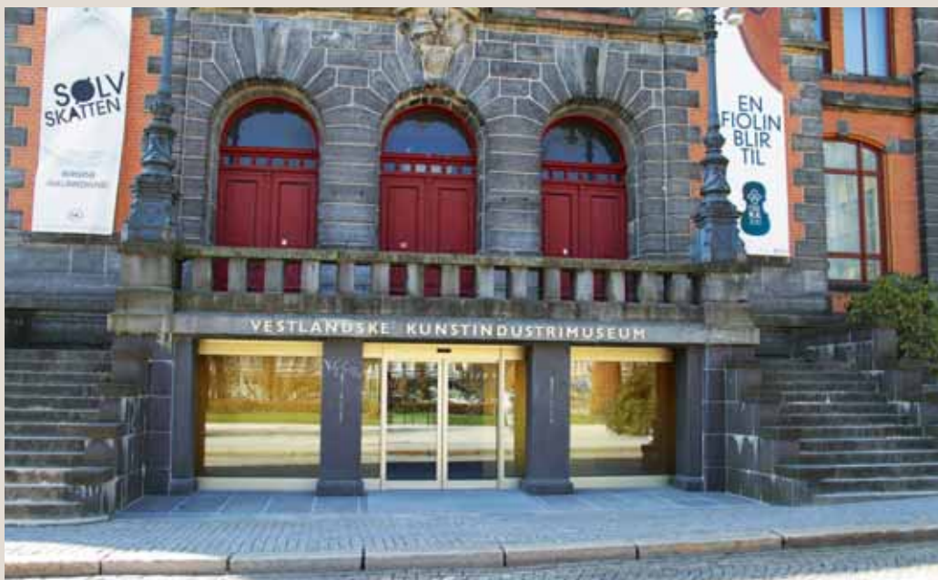
Part of the main facade with changes made to the main entrance – better lighting, glass doors with a photo-cell mechanism and information boards adapted to suit those who are vision impaired. Photo: Bergen municipality
