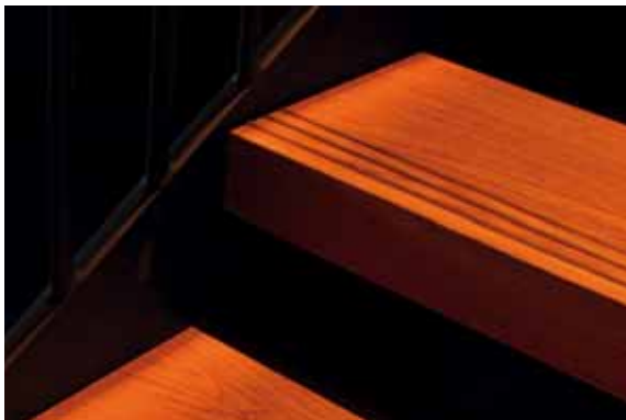
Contrasts between the steps and risers help to make the stairs visible. A brass strip marks the front of the step.
