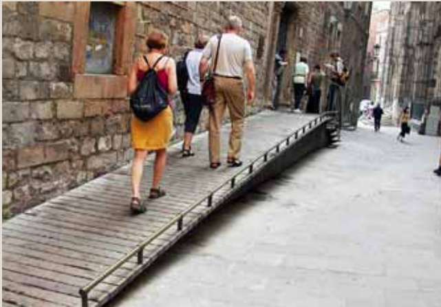
Ramp, Barcelona. The ramp is designed so that it can be dismantled without damaging the building.
