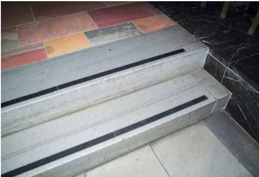
Marked steps. A line of coloured material has been cut into the outer part of the step.
