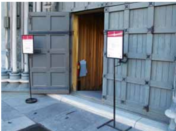
The main entrance on the western side. 10cm difference in level between the ground and church floor. Ramp just inside the door.
